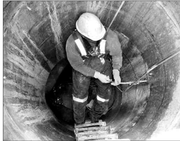
Manhole joint injection.
